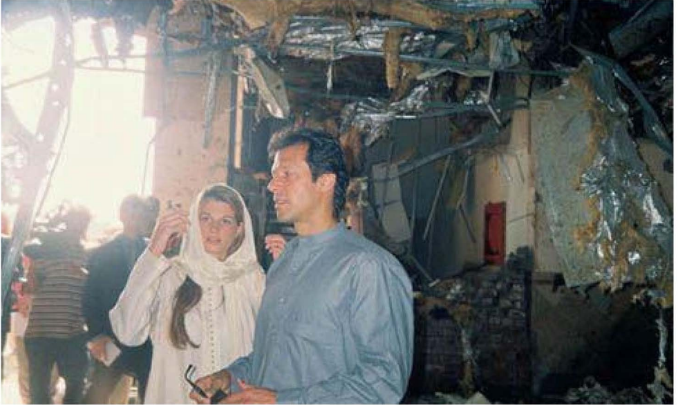
The hospital was bombed in 1996. Jemima and I inspect the damage.
