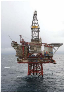
Figure 19.4 An Exxon Mobil oil platform in the North Sea
